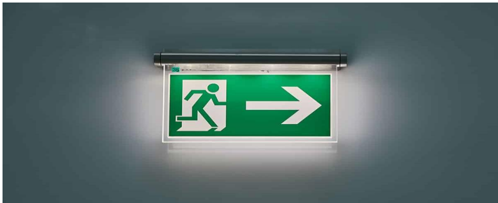
Figure 9.5: Emergency Lighting Signs
