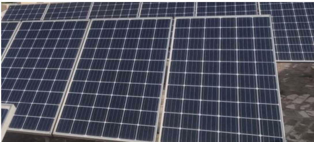
Energy efficient inverters (Combined Cooling Heating and Power Integration Unit)
