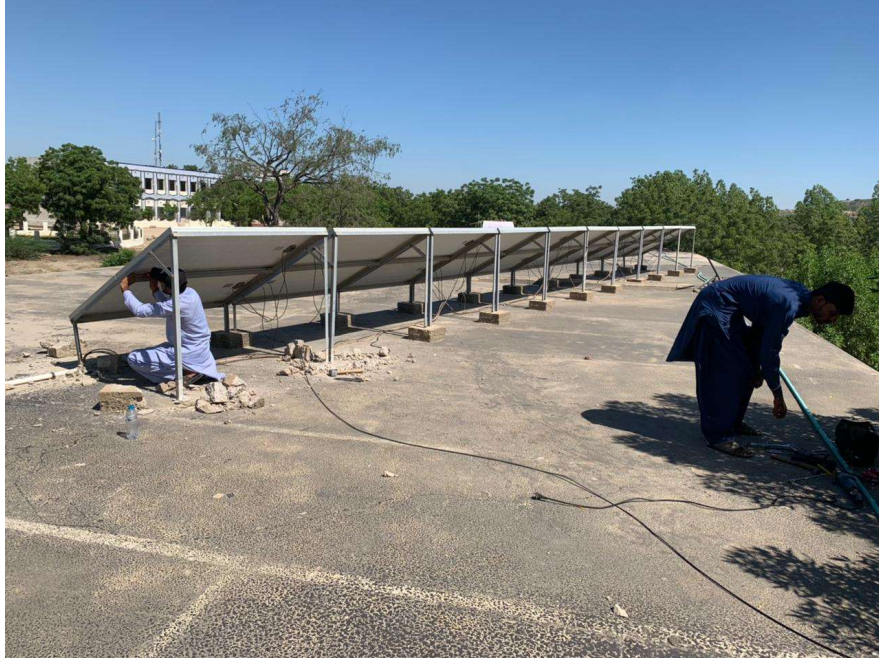
Solar Panels installation
