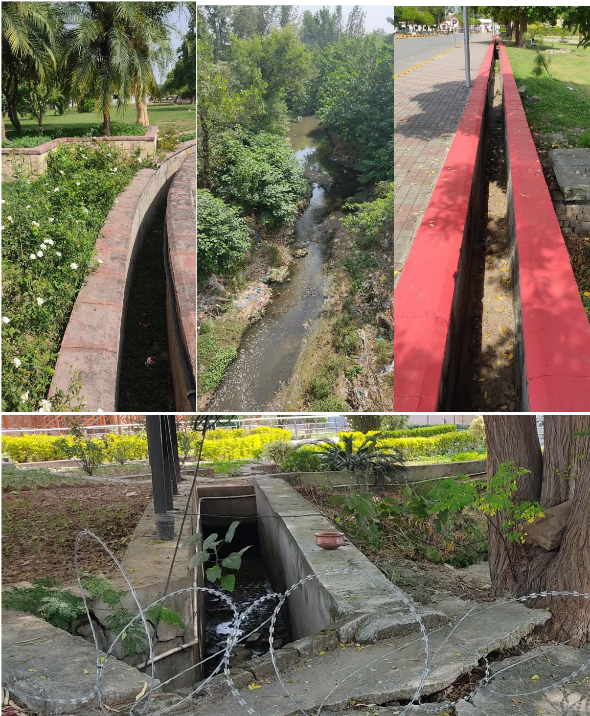
Water canals have been constructed to conserve rainwater and used water
