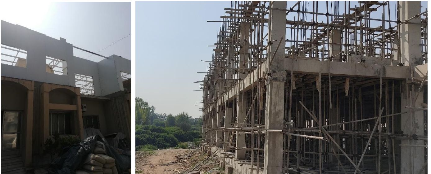
Treated water is used in construction
