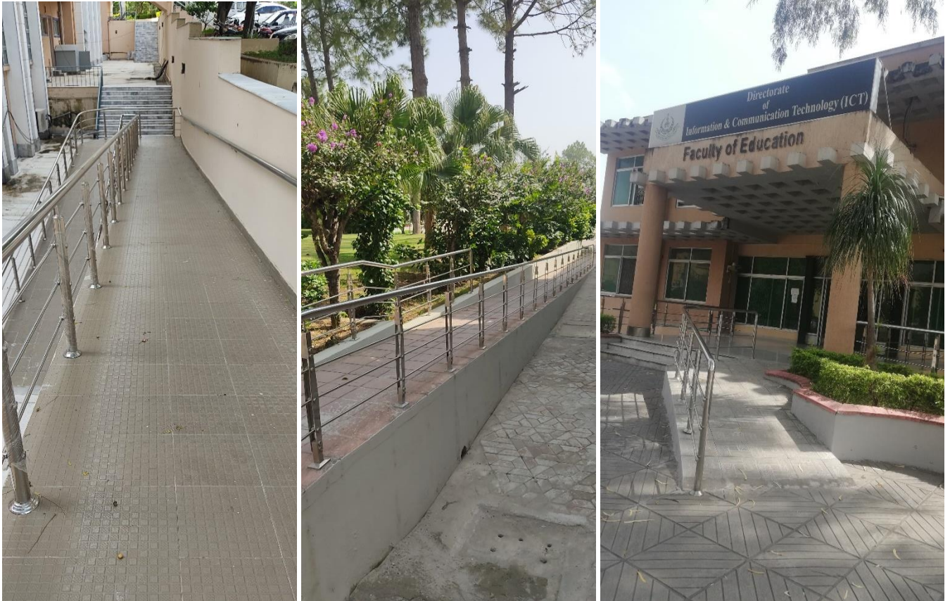
Wheelchair Ramps at entrance of all buildings
