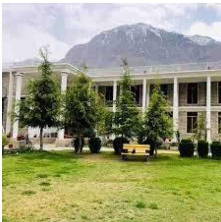
Gilgit campus construction work
